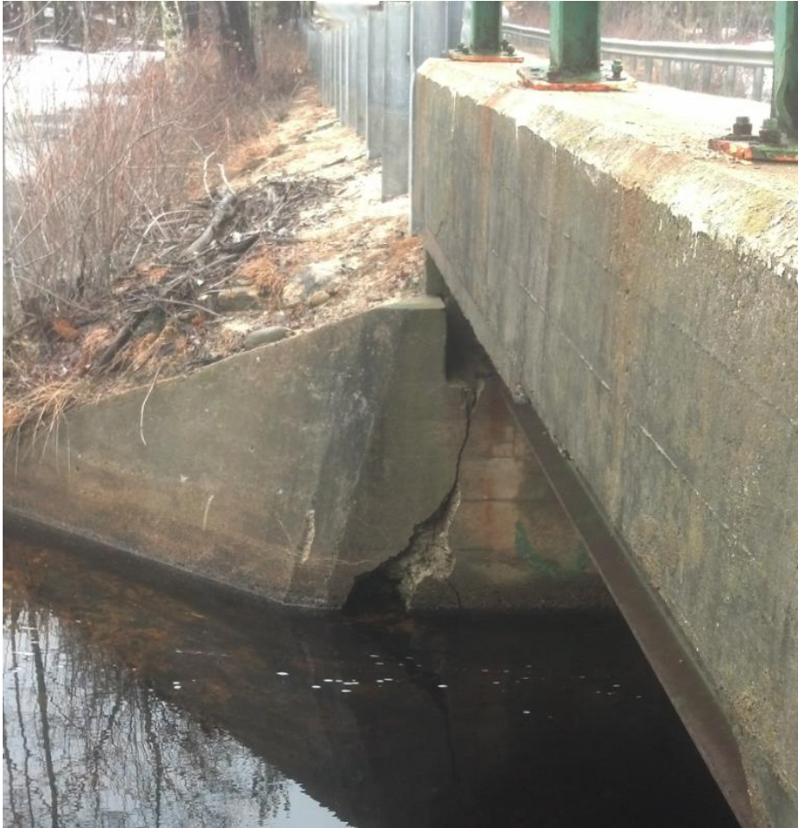
Large Crack & Spalling in Abutment
