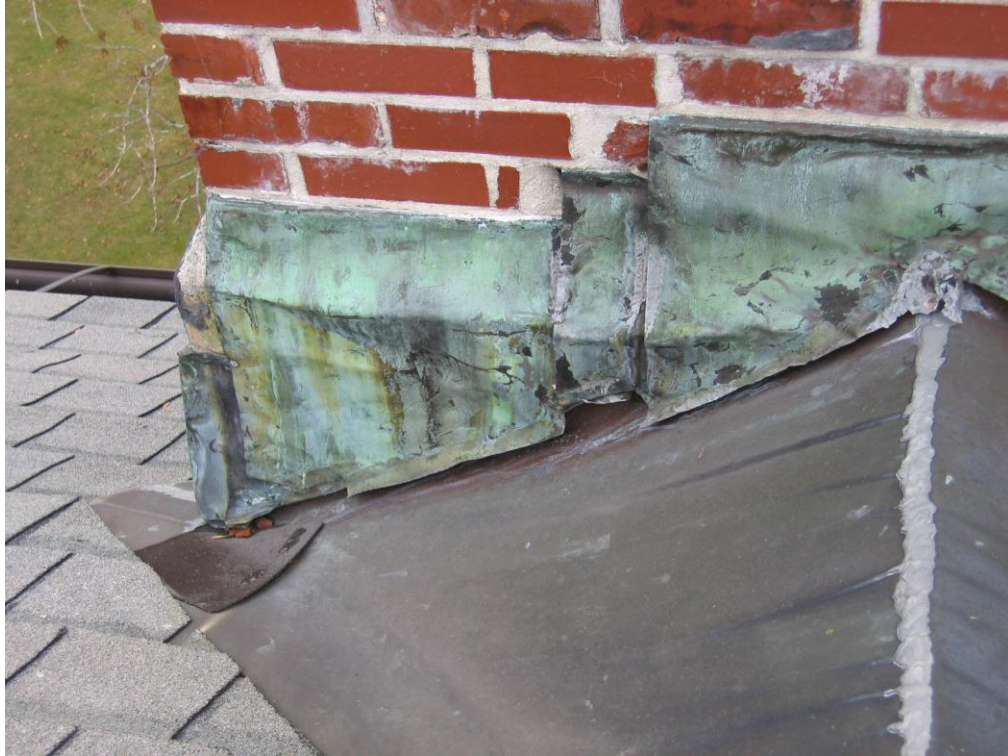
Cricket covering in copper is good, counterflashing on chimney is original and is serviceable. Object on left is a shingle, not damage to the copper.
