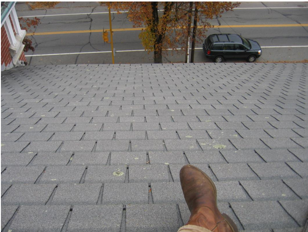
Roof on front of building is still serviceable
