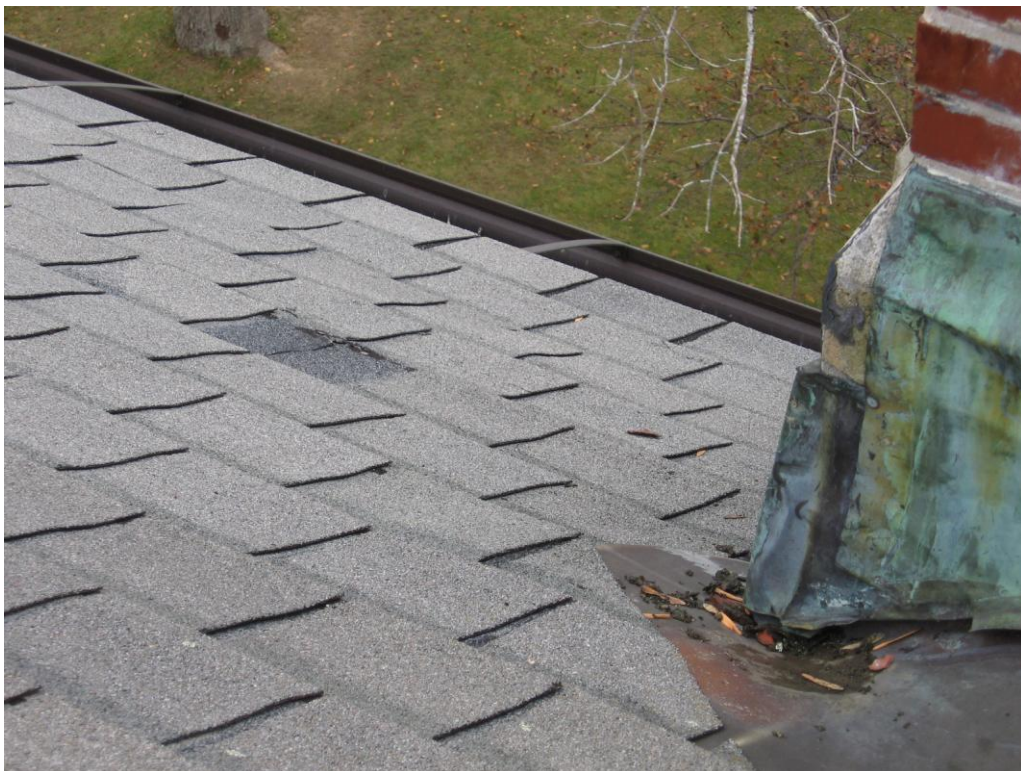
Shingle is also missing towards the front of the building near chimney
