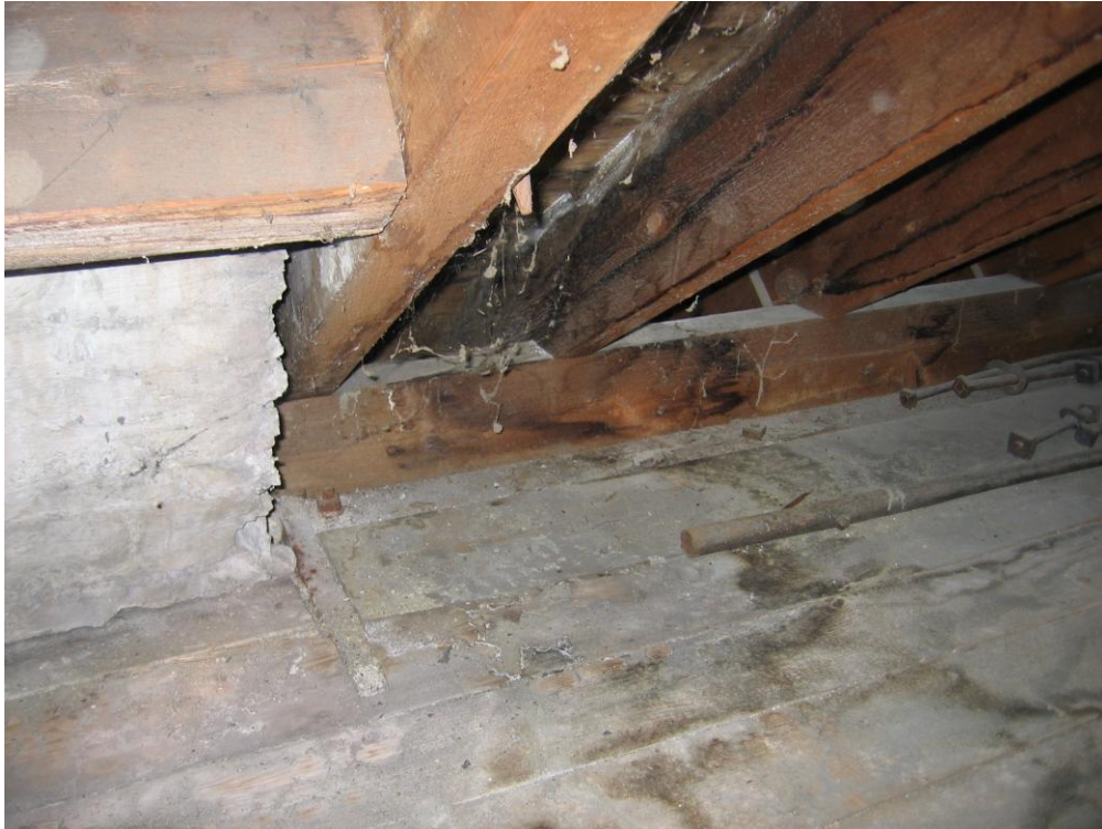
South chimney from attic showing water stains
