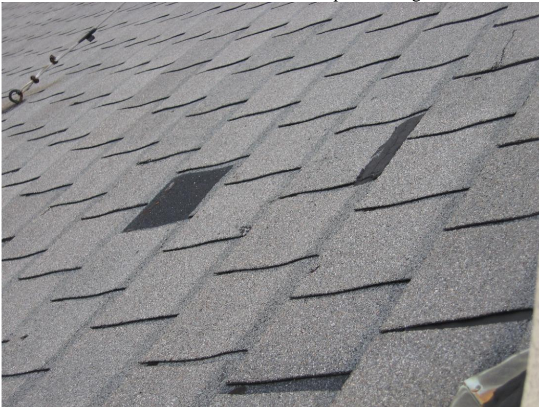
Damaged shingle or two near curb on rear slope.
