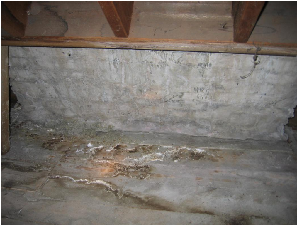
South chimney – attic water stains
