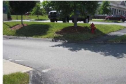
Poorly defined crosswalk
