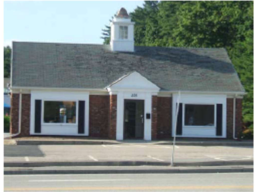
Front yard with no landscaping
